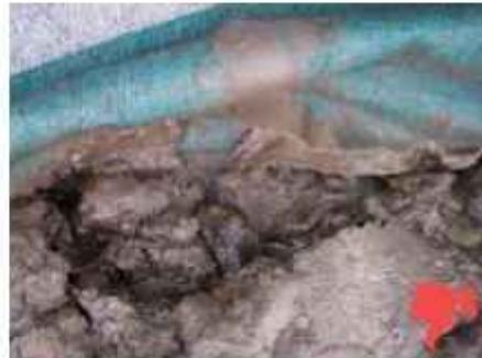
Not buried deep enough & ground poorly compacted.
