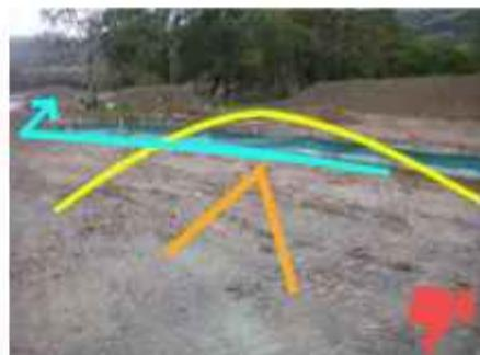
Runoff follows the fence line making erosion worse.
